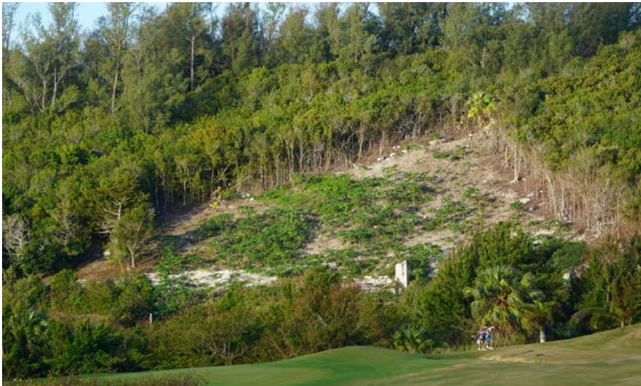
This cleared hillside at Judkin Lane is now being quarried
